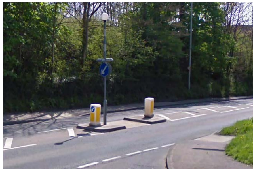
Figure 12 Uncontrolled pedestrian crossing point
